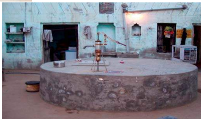
Figure 2.30: Small cylindrical underground well (tanka)
