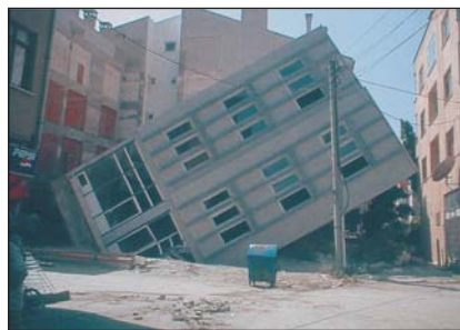
Tilting of building due to liquefaction (Adapazari, Turkey 1999) By Bachmann H., Sesimic Conceptual Design of Buildings
